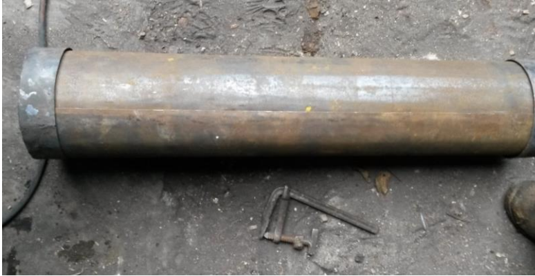
Figure 31: Lids used to hold the rolled plate before welding.
