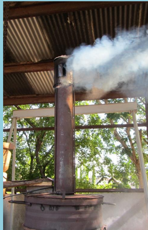
Figure 57: White colour leaving the chimney
