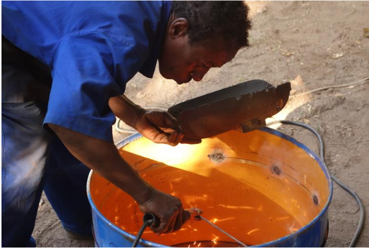
Figure 11: Welding the upper and lower part
