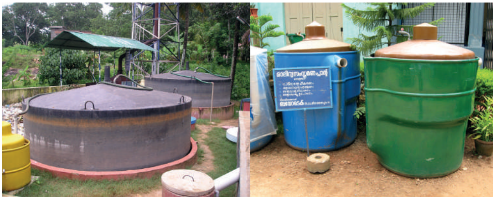
Figure 14: Underground floating-drum digester for market waste in India (left) and above ground floating-drum digester for households in India, made of fiberglass reinforced plastic (right)
