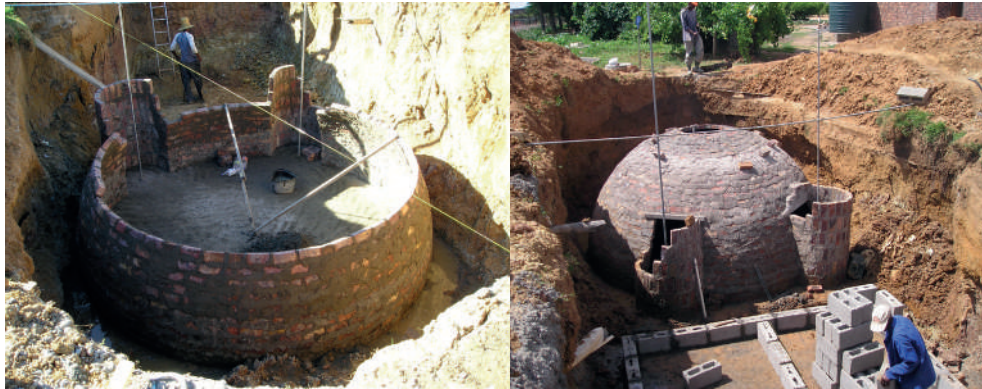
Figure 11: Fixed-dome digester under construction in Lesotho
