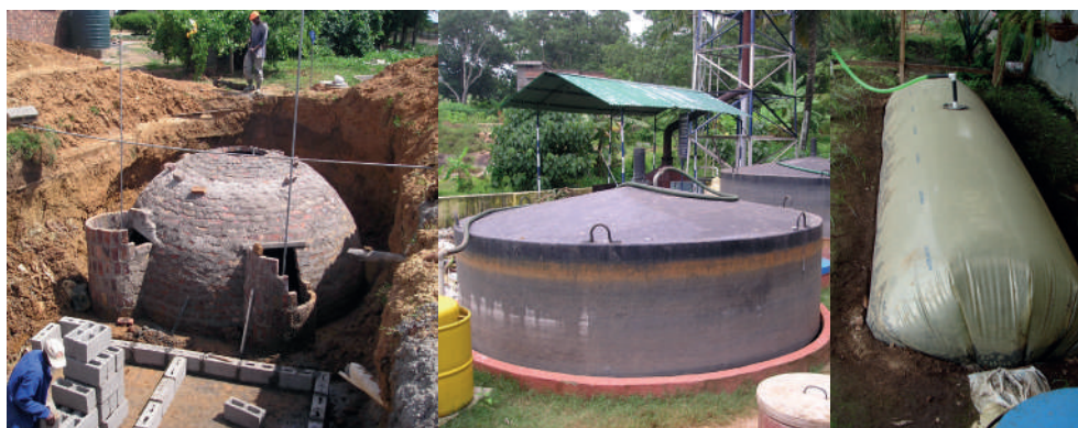
Figure 9: Different anaerobic digesters. A fixed dome digester under construction; a floating dome digester and a balloon digester, from right to left.
