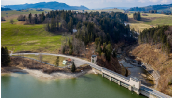
The Sihlsee dam is part of the Etzelwerk pumped storage power plant. (Photo: Alessandro Della Bella, Eawag)
