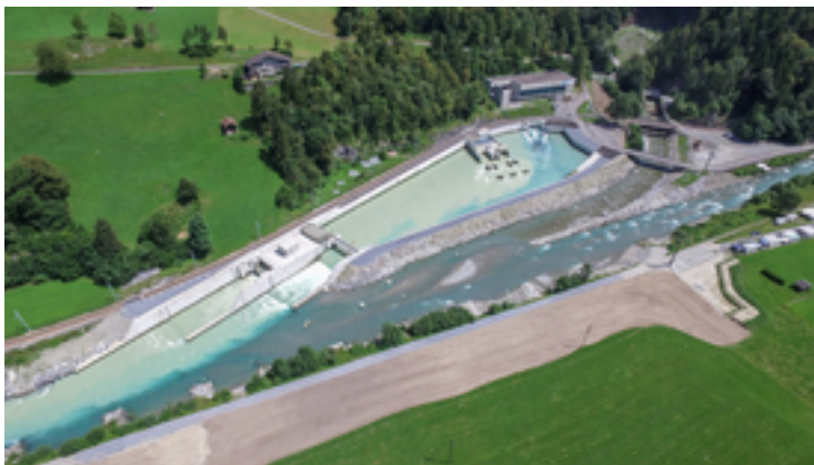
A calming basin reduces the negative ecological effects of hydropeaking in the Aare river near Innertkirchen. (Photo: Markus Zeh)
