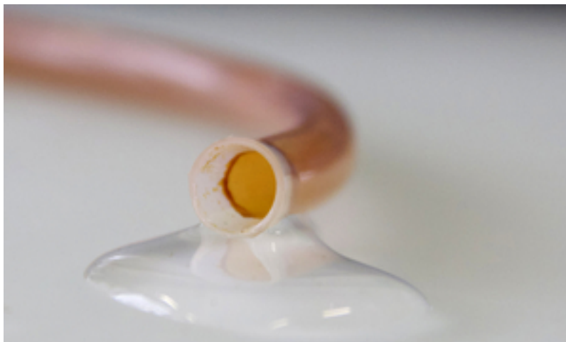
This plastic tube inside a shower hose is coated with a brownish, iron-containing biofilm.
