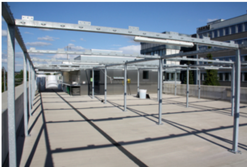
Accessible roof for open-air experiments, with construction to shade the equipment. Photo: Andri Bryner, Eawag
