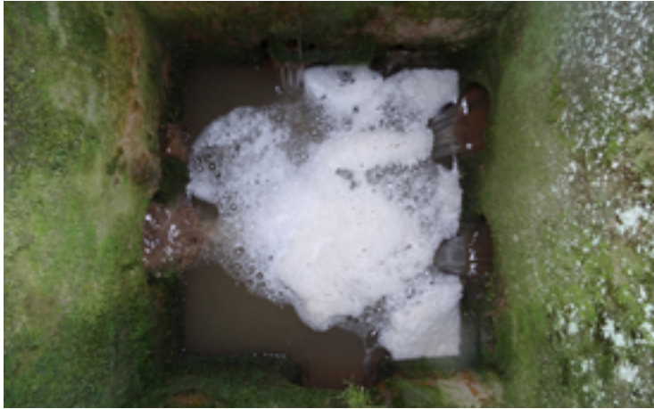
Here, water from several inlet shafts converges before flowing directly into the nearby stream. (Photo: Eawag, Urs Schönenberger)
