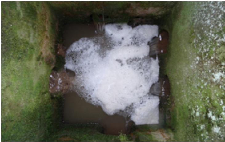
Here, water from several inlet shafts converges before flowing directly into the nearby stream. (Photo: Eawag, Urs Schönenberger)
