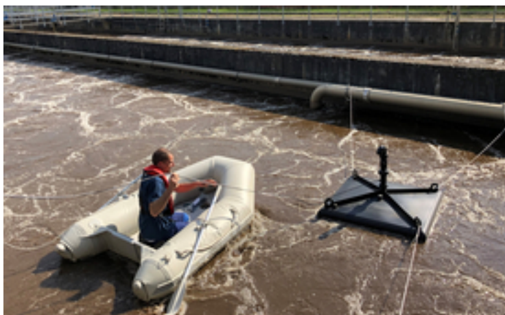
Eawag researcher Wenzel Gruber undertaking some maintenance work on the measurement system at the Moossee Urtenenbach WTP. (Photo: Andrin Moosmann)
