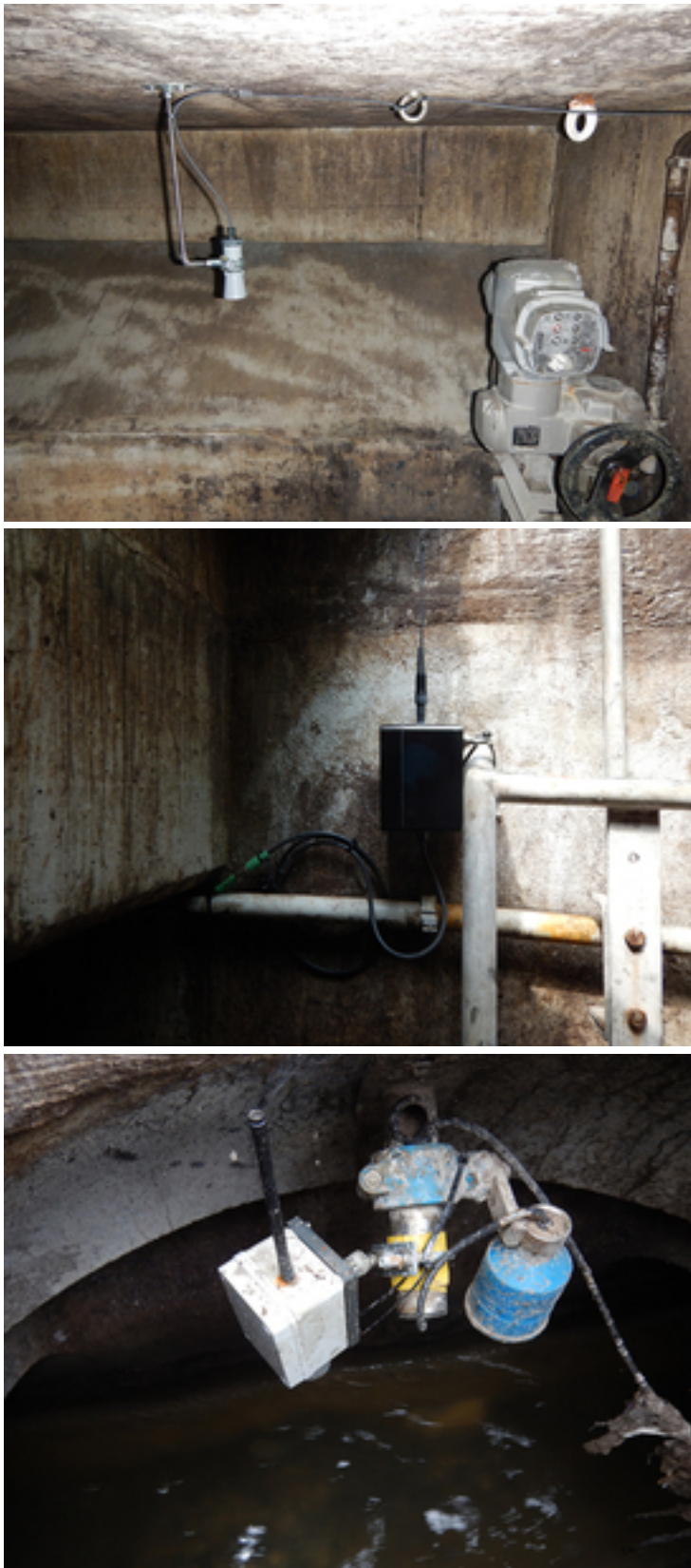
Fig. 2: The wireless sensors transmit spatially and temporally high-resolution measurements of drainage and water levels to the researchers.
