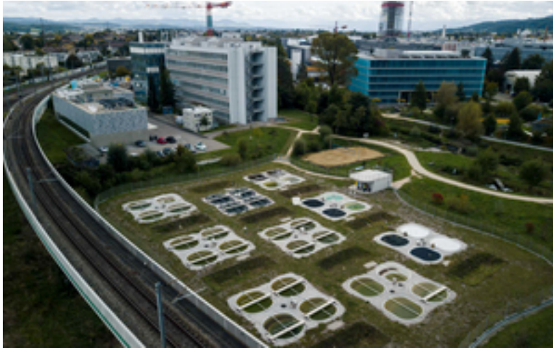
The pond facility at Eawag. (Photo: Thomas Klaper)
