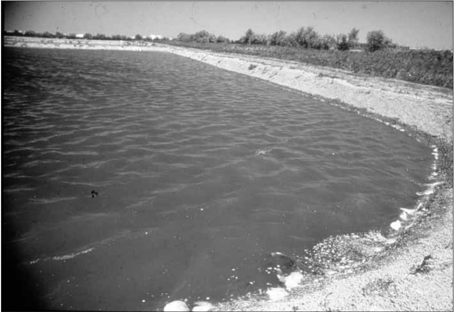
Figure 13.3 Embankment Protection by Stone Rip-rap
