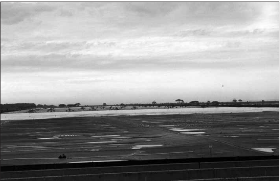
Figure 13.12 Covered Anaerobic Pond at the Western Treatment Plant, Melbourne, Australia
