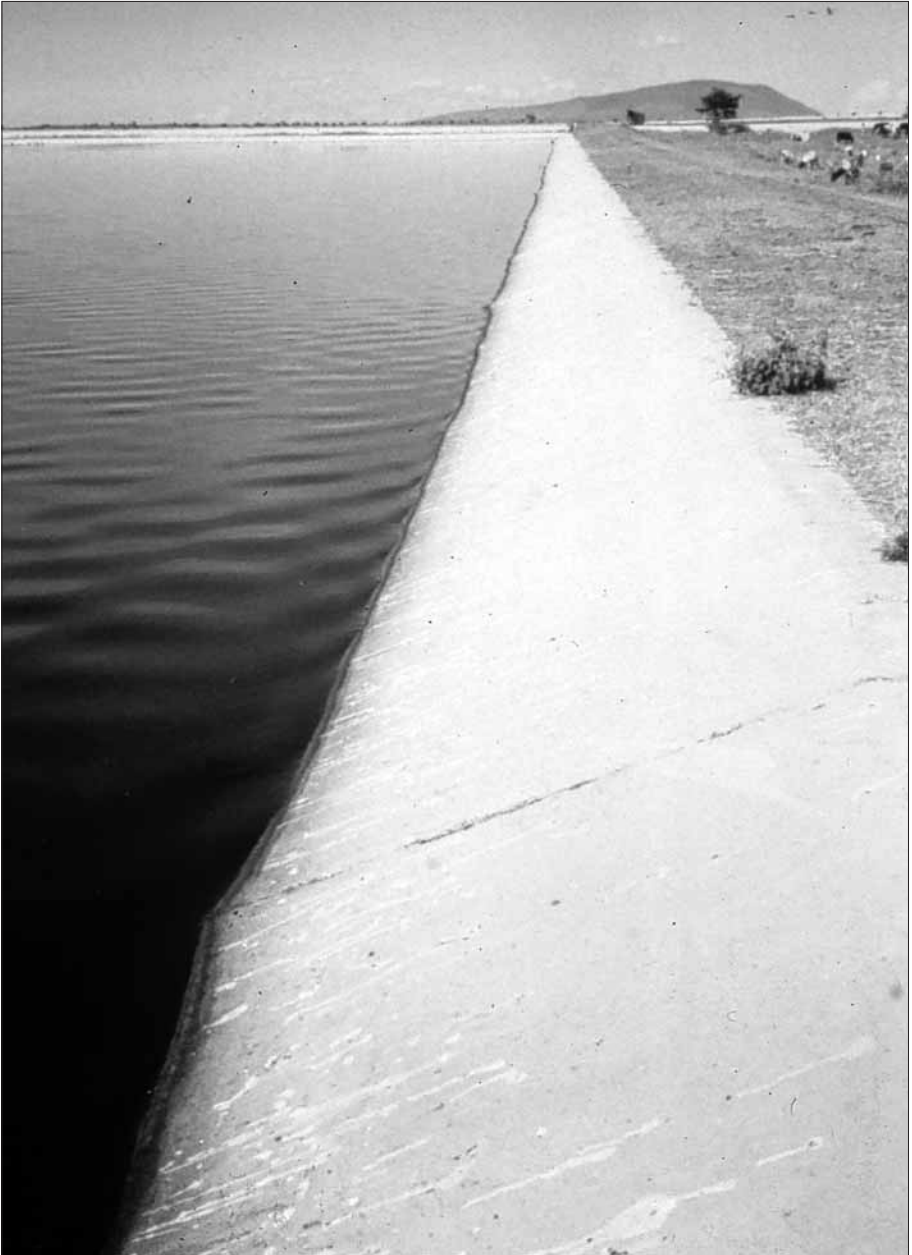
Figure 13.1 Embankment Protection by Concrete Cast in situ
