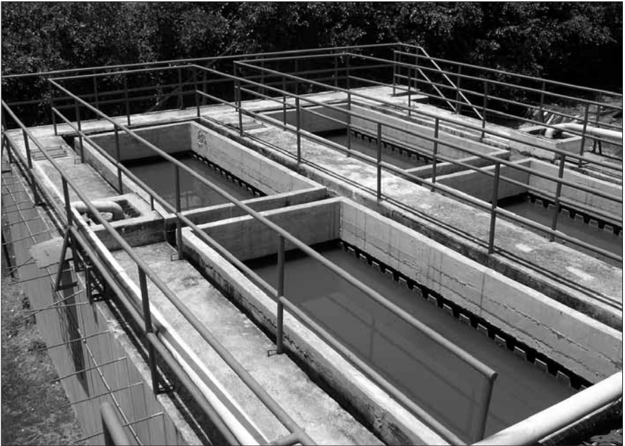
Figure 18.1 An UASB at Ginebra, Valle del Cauca, Southwest Colombia, Treating 10 l/s of Domestic Wastewater
