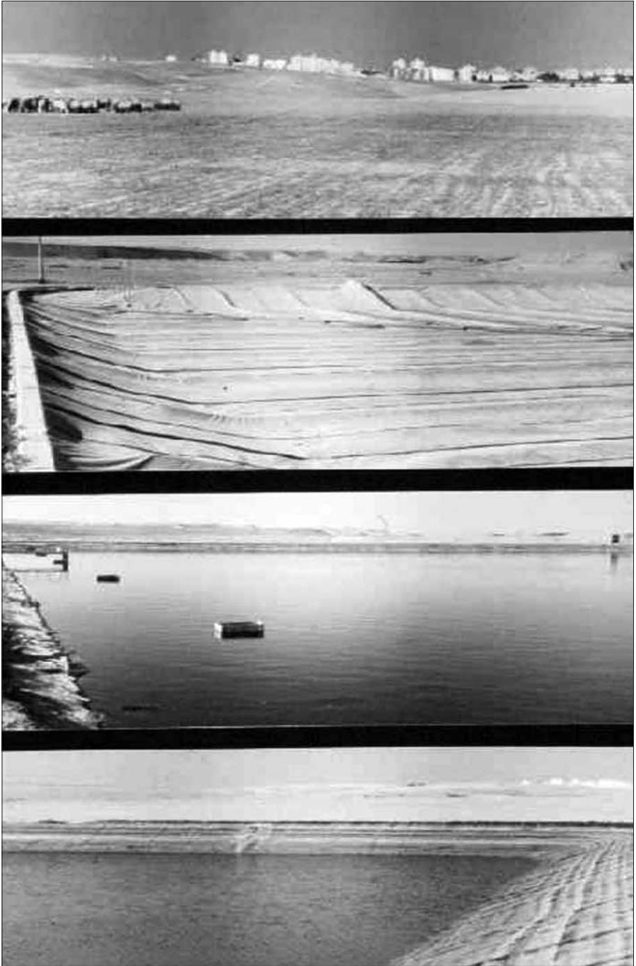
Note: (a) view of Arad town in the Negev desert, (b) covered anaerobic pond, (c) WSTR in rest phase, and (d) WSTR in use phase.
