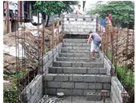
Figure 14. Anaerobic baffled reactor under construction.
