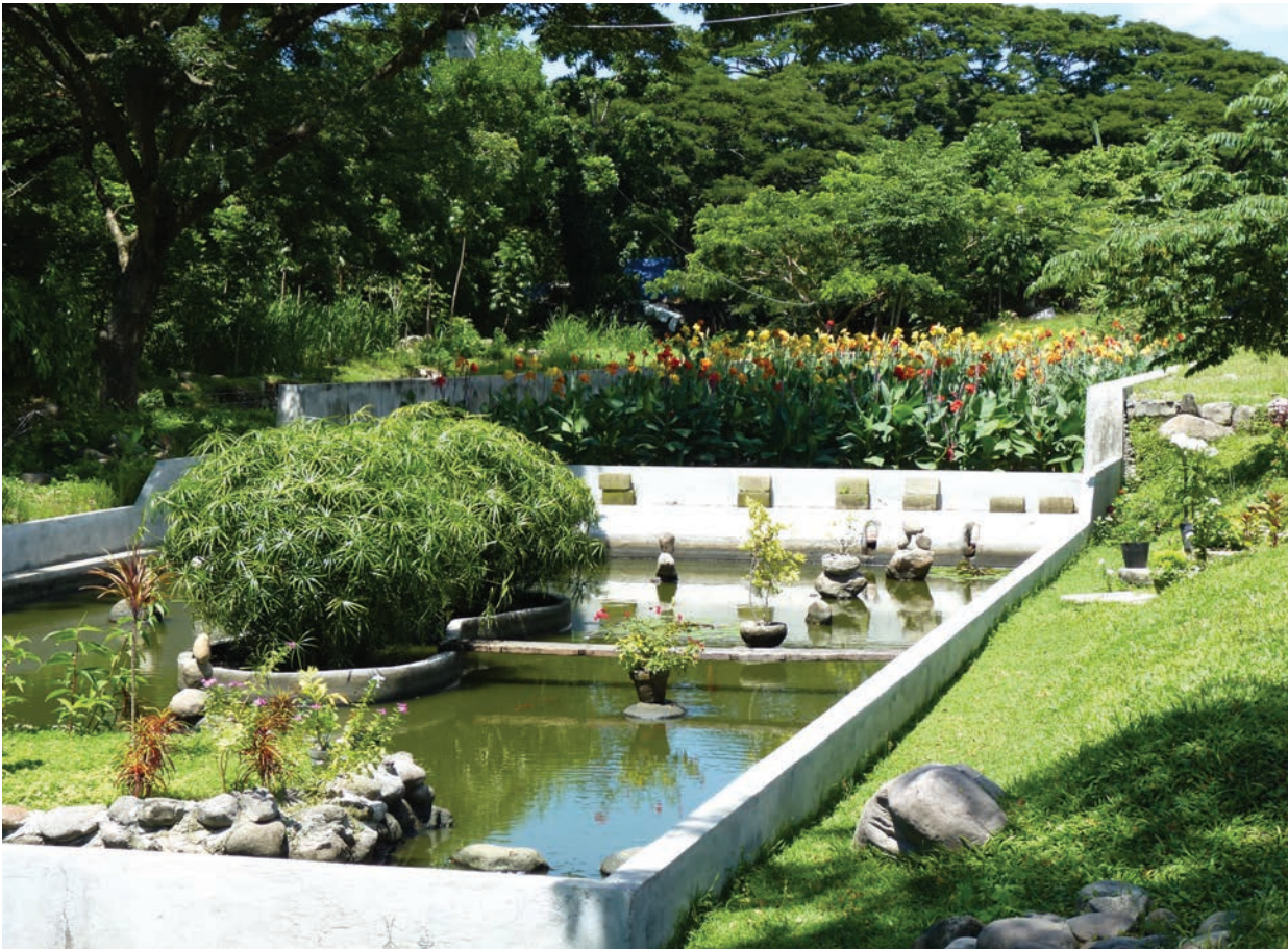
Figure 17. This natural disinfection pond at Dumaguete City's septage treatment facility serves as an indicator pond where fish are used to demonstrate the purity of the water.
