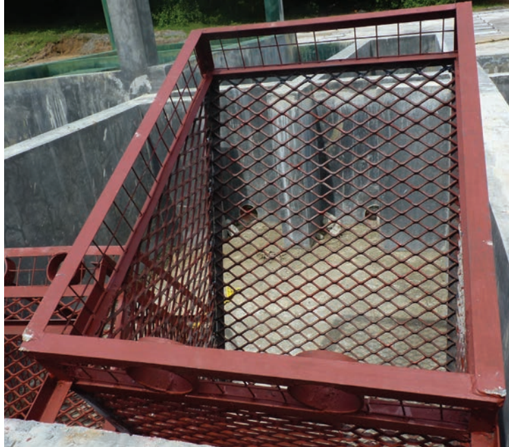
Figure 6. Trash rack constructed out of painted metal. Hinged at one end, the racks are easy to tip collected debris into conveniently located trash bins.
