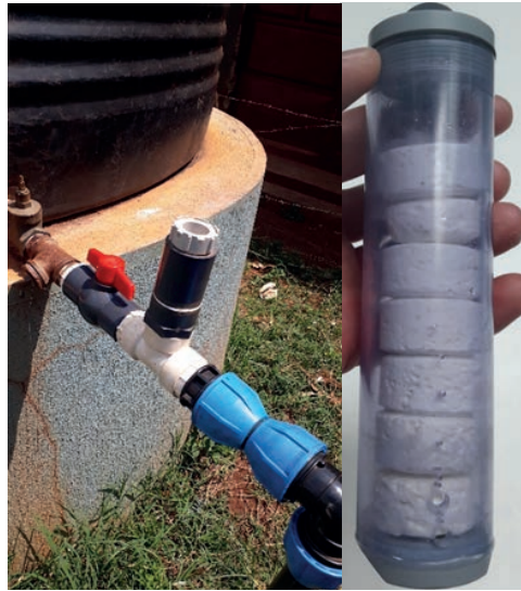
Figure 67: T-chlorinator and cylinder
