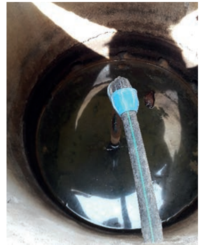
Figure 15: Inside of the infiltration well made from cement rings
