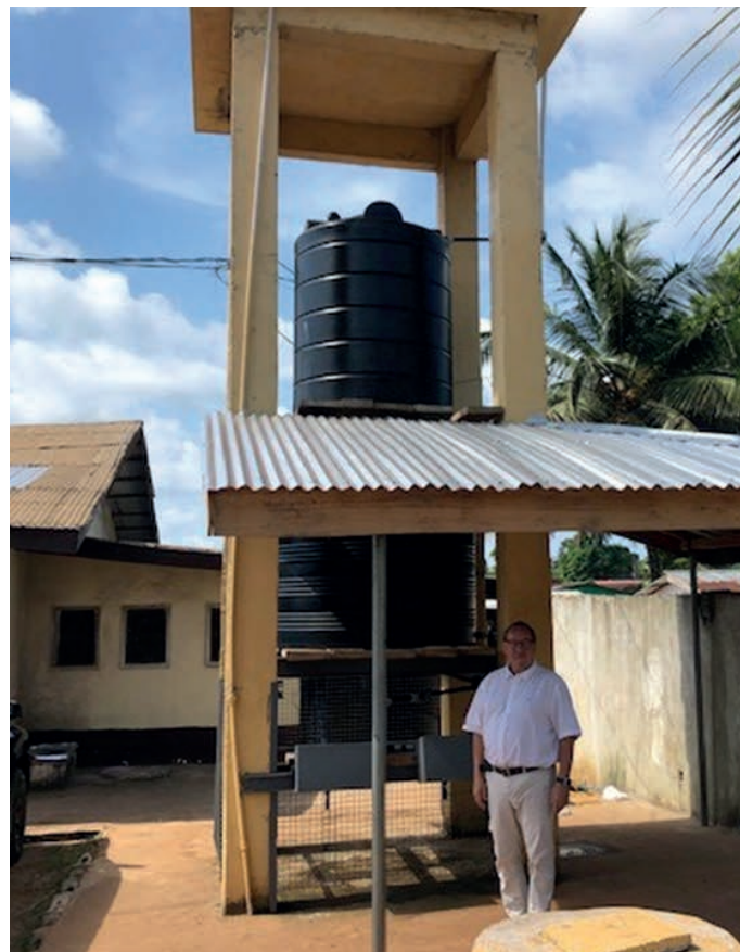
Figure 40: Picture of vertical GDM treatment system
