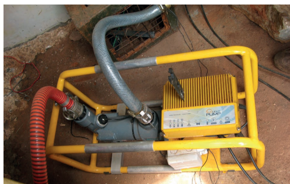
Figure 20: Ennos Sunlight pump installation
