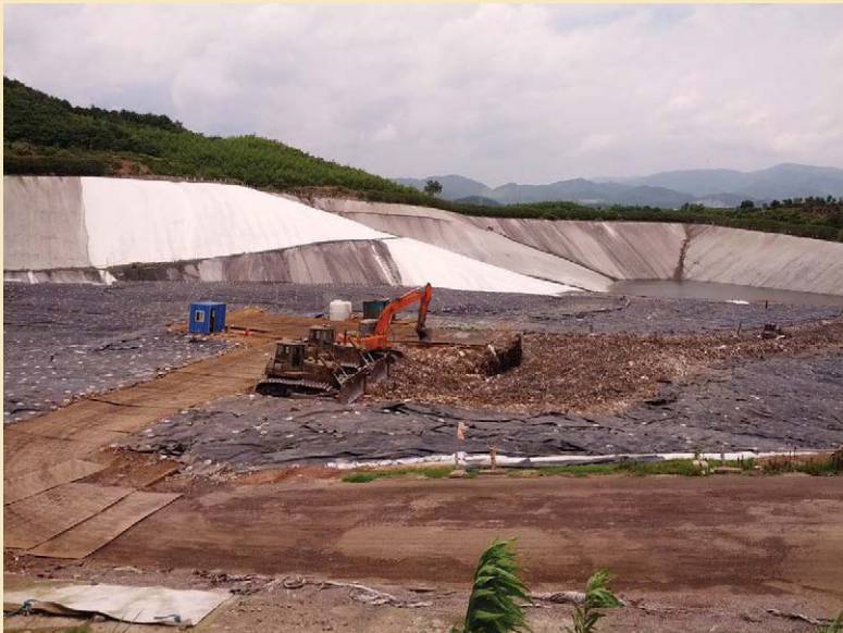
Photo 3.1 Landfill in China
