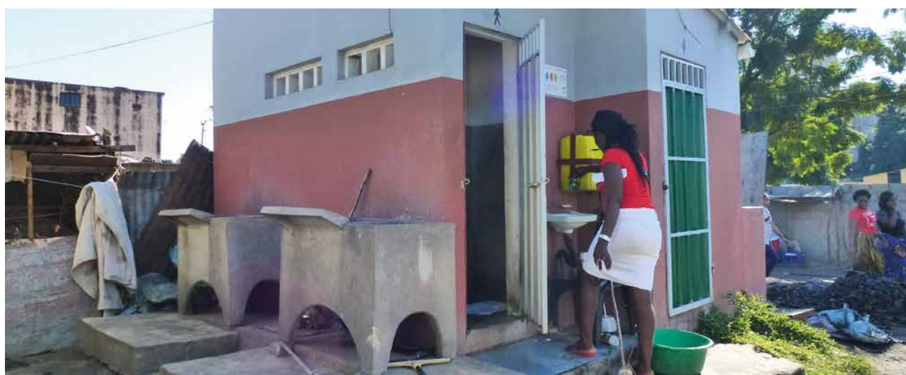
A communal sanitation block in Chamanculo, Maputo, Mozambique.
