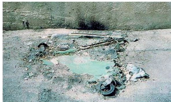
c) This was a 1,100 litre green plastic bin until someone put hot ashes into it. Alternatively, someone may have set its contents on fire because it had not been emptied or for some other reason.
