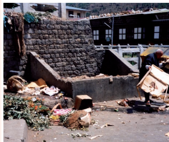
b) Community bunker (compound); difficult to empty
