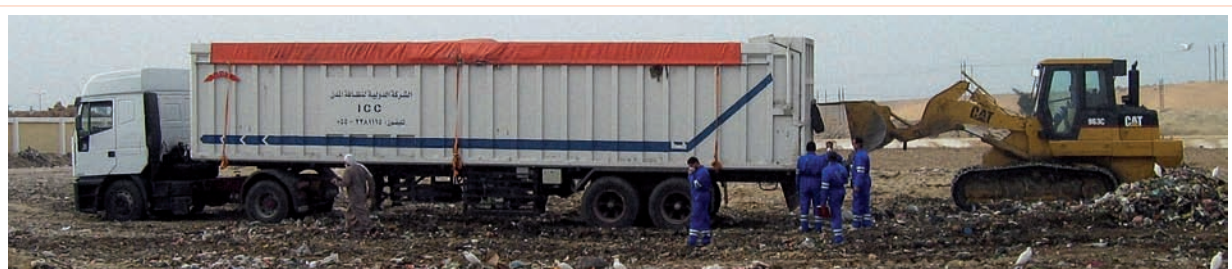
Photo 8.4 Tracked loader helping an empty articulated truck to move off the waste
