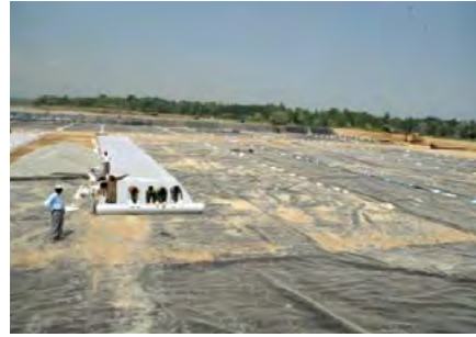
Overlaying the HDPE Liner
