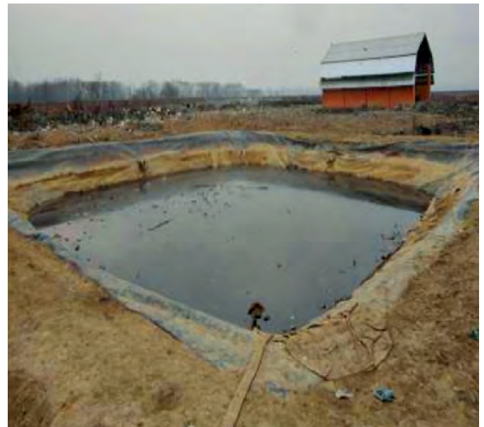
Leachate collection pond
