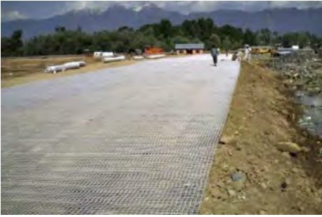
Laying of geogrid
