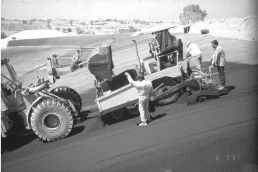
Photo 3.6 Asphalt liners for a sanitary landfill
