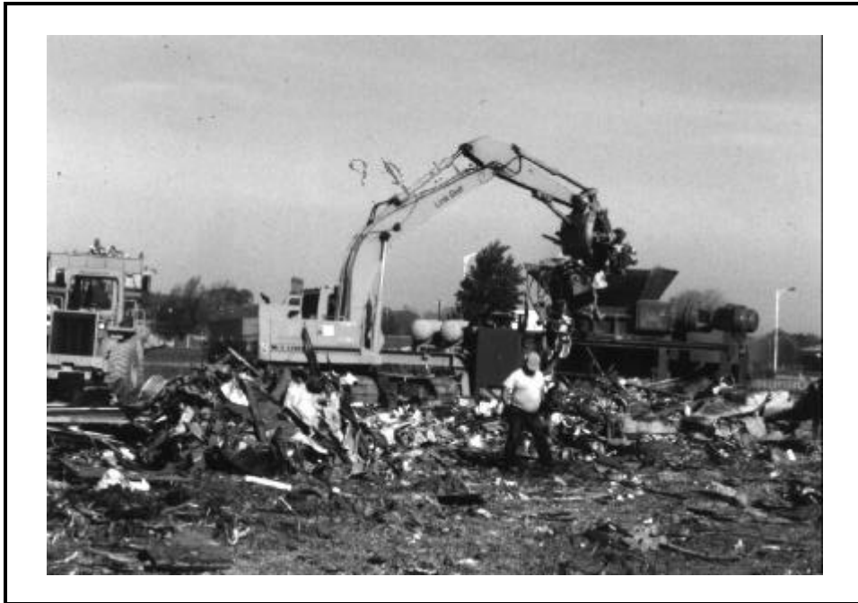
Figure 12. Demolition debris being loaded into debris compactor.
