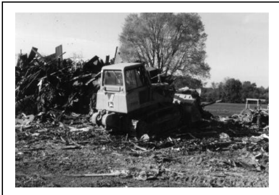
Figure 1. Heavy equipment being used to smash and compact building material.
