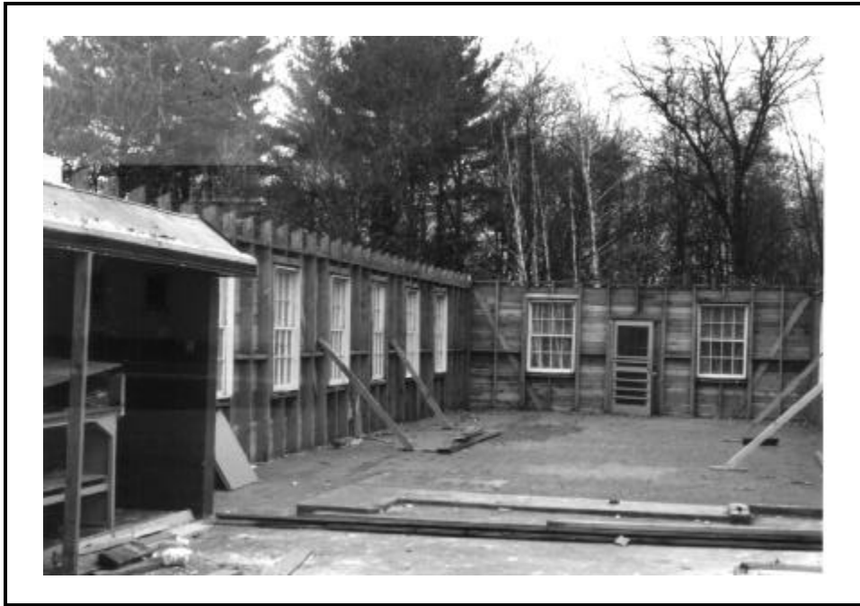
Figure 6. Wood-framed barracks in process of deconstruction.
