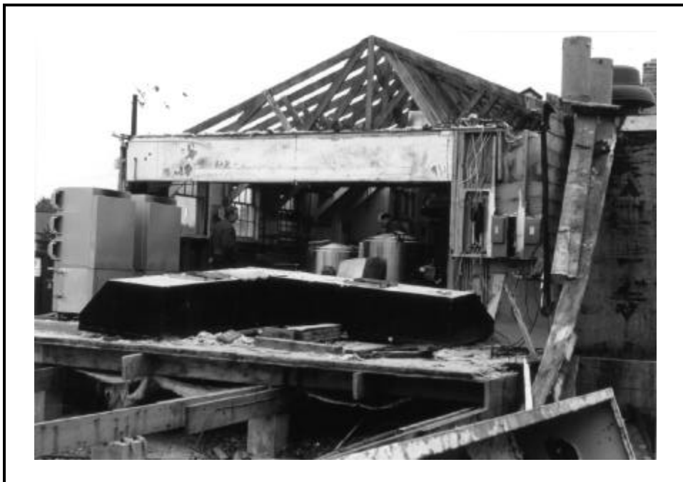
Figure 7. Wood-framed mess hall in process of deconstruction.
