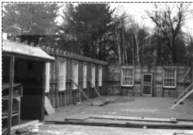
Wood-framed barracks in process of deconstruction.
