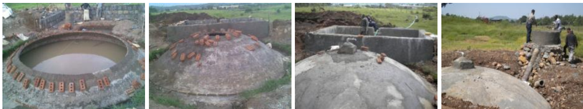
Figure 14: Construction of biogas digester (left two pictures by G.Alemnew)
