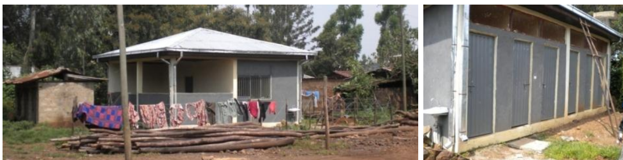
Figure 35: LEM Ethiopia Integrated sanitation facility in kebele Gish Abay. Left picture: New sanitation facility with old latrine (left) and AD system (right of the building). Right picture: Showers and toilets
