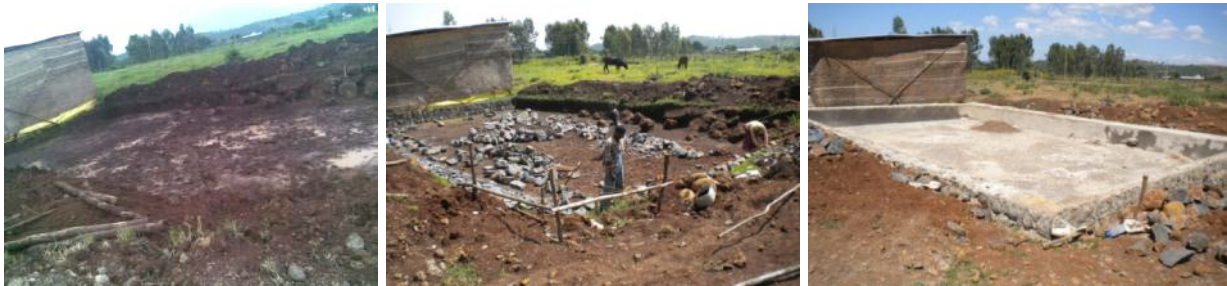
Figure 15: Construction of composting pit (left picture by G.Alemnew)
