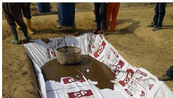
Figure 18: An infiltration bed lined with cut-open sand bags (source: Bangladesh Red Crescent & British Red Cross, 2023)
