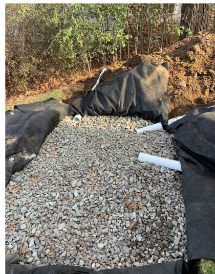
Figure 22: Infiltration trench (Deer Lake Conservancy, n.d.)
