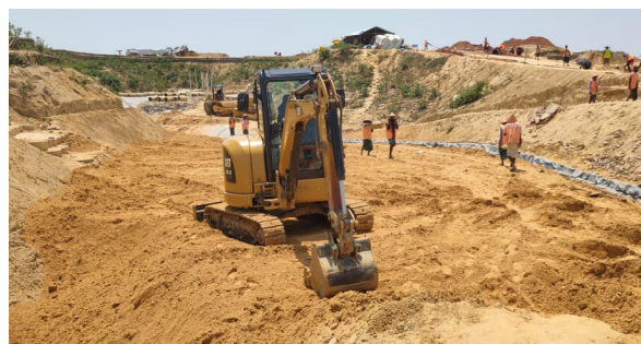
Figure 15: Landfill preparation in Cox's Bazar: excavator preparing the clay bottom liner (photo credit: UNDP)
