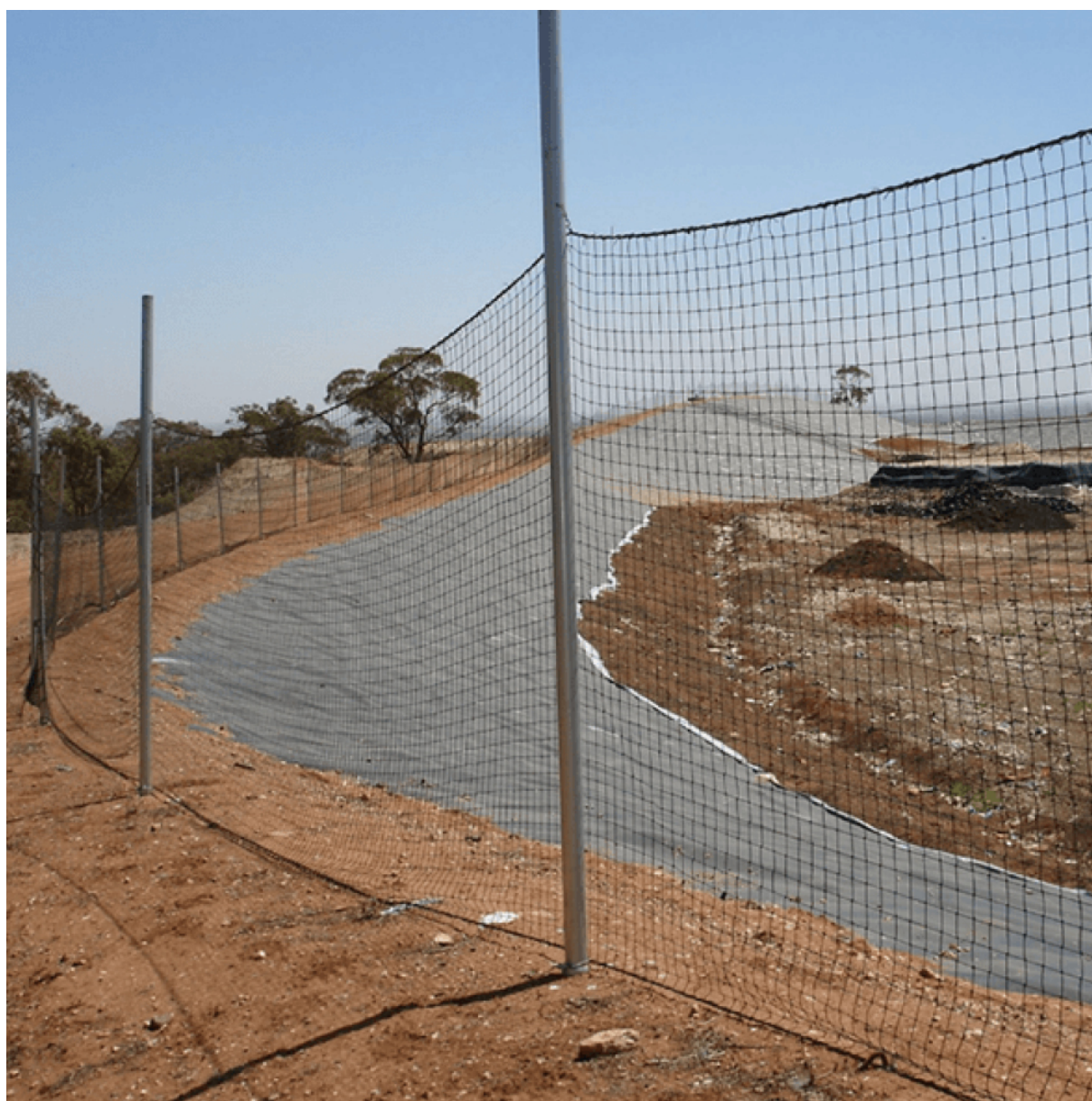
Figure 17: Fence to stop windblown waste from getting out of the disposal site (Quins, n.d.)
