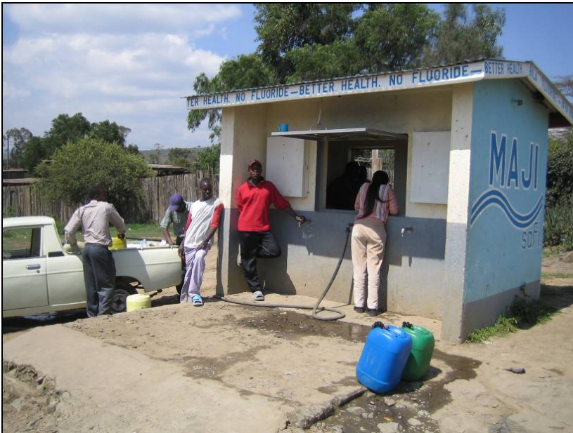
Figure 6-2: Water kiosk in Naivasha that sells defluoridated water from a community filter installed by CDN WQ. The water kiosks are opened at fixed times that are set by the local water management.
